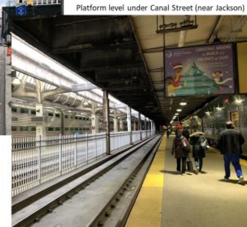
Platform level under Canal Street (near Jackson)
